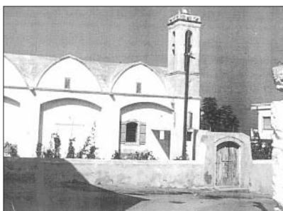
The church of Ayios Epiktitos in Ayios Epiktitos village. The Cross is cut by the Turks, the windows opened and the whole condition of the church and the yard is very bad. Recently, the church has been converted into a Muslim Mosque. This is only one of the many destroyed constantly and systematically by the Turkish forces.
