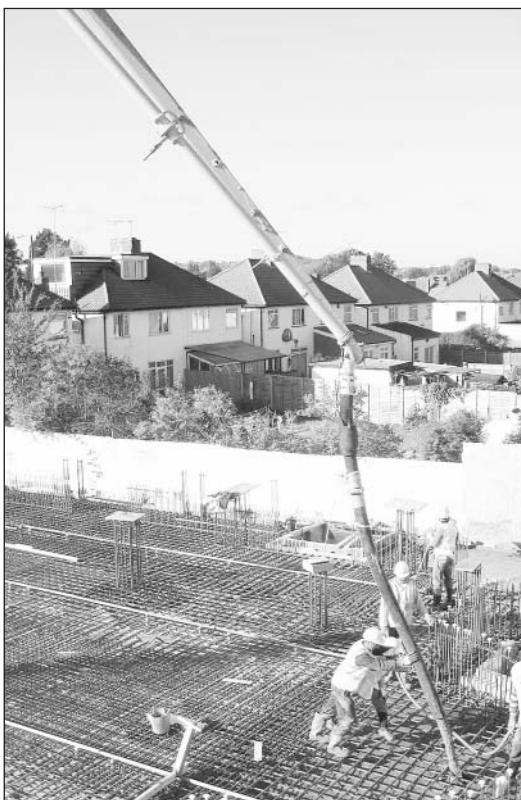
CONSTRUCTION WORKS AT THE HARROW SITE HAVE ALREADY STARTED TAKING PLACE
